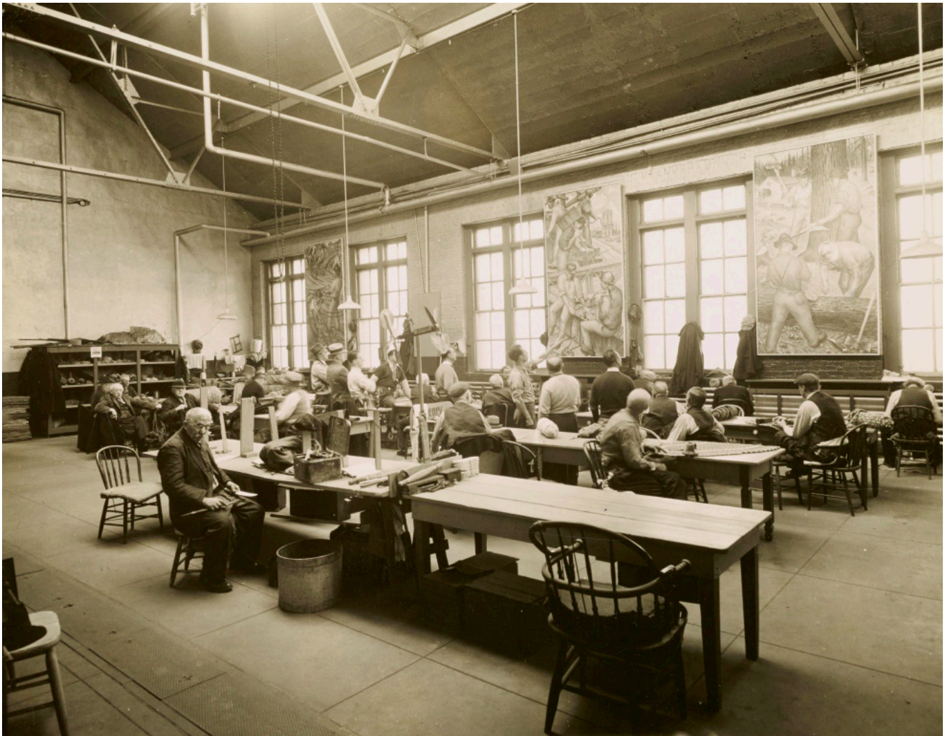
WPA murals inside the Farm Colony's Laundry Building | Photo courtesy of Vengoechea + Boyland Architecture/Urban Planning via NYC Municipal Archives
