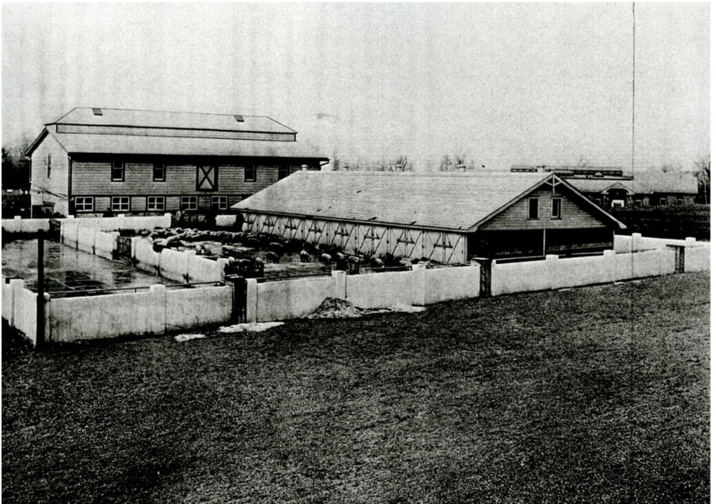
Farm Colony piggery and vegetable house, 1914 | Photo courtesy of Vengoechea + Boyland Architecture/Urban Planning via NYC Municipal Archives
